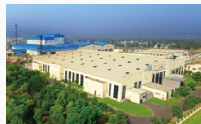
IJL Bawal Plant
