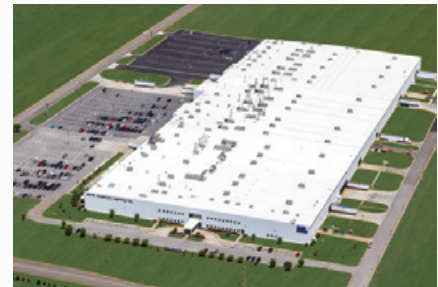
NAL Alabama Plant
