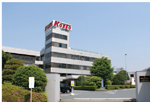
KI HOLDINGS CO., LTD. Head Office and Plant
