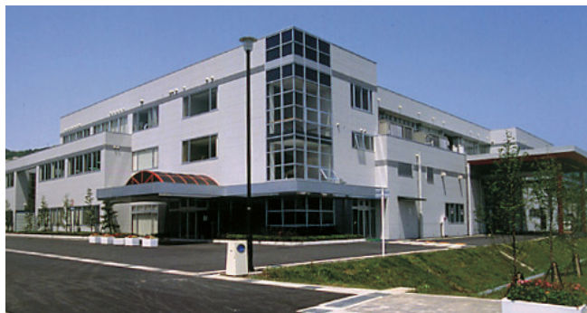
KOITO MANUFACTURING Fujikawa Tooling Plant
