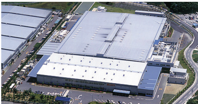
KOITO MANUFACTURING Sagara Plant
