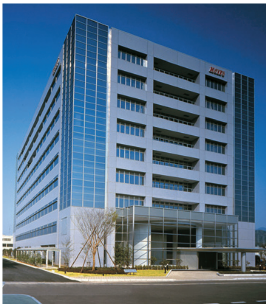
KOITO MANUFACTURING Technical Center
