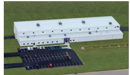
NAL Indiana Tooling Plant
