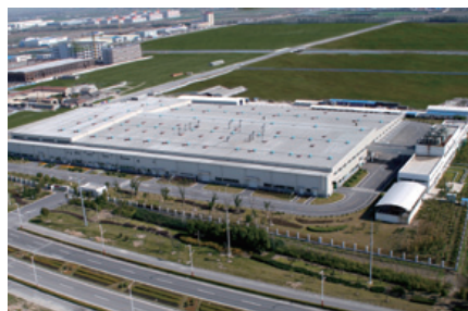
Shanghai Koito Third Plant
