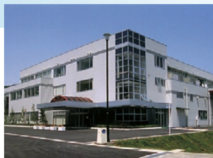
KOITO MANUFACTURING Fujikawa Tooling Plant
