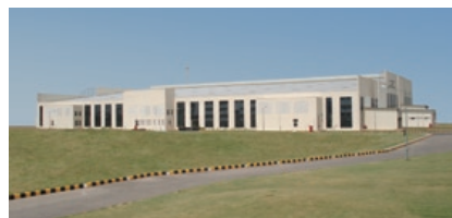
IJL Bawal Plant
