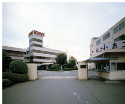
KI HOLDINGS CO., LTD. Head Office and Plant
