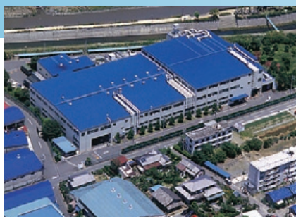
KOITO MANUFACTURING Kikkawa Plant
