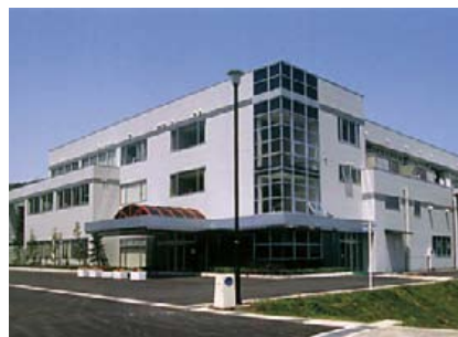
KOITO MANUFACTURING Fujikawa Tooling Plant
