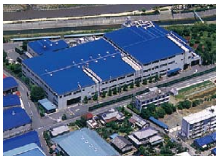
KOITO MANUFACTURING Kikkawa Plant
