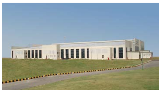
IJL Bawal Plant
