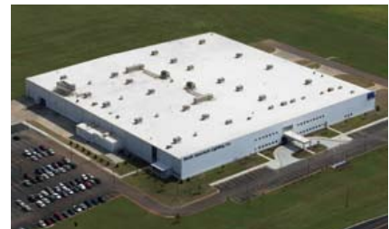
NAL Alabama Plant
