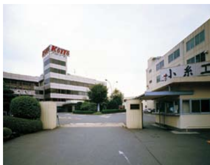
KOITO INDUSTRIES, LIMITED Head Office and Plant
