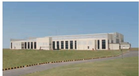
▶ IJL Bawal Plant
