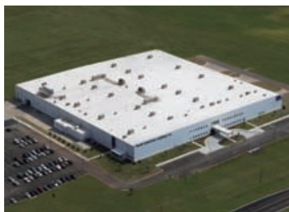
▶ NAL Alabama Plant
