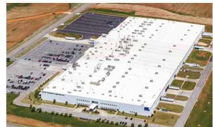
NAL Alabama Plant
