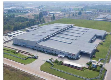
THAI KOITO Prachinburi Plant
