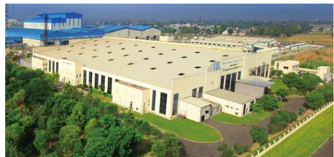
IJL Bawal Plant
