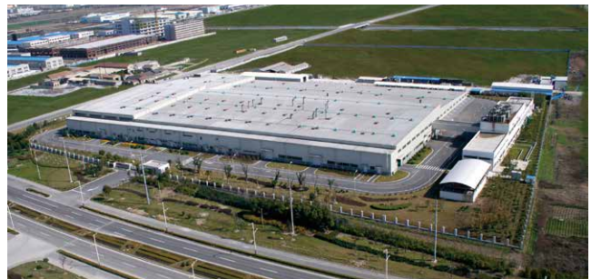
Shanghai Koito Third Plant
