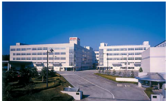
KOITO ELECTRIC INDUSTRIES Head Office and Fuji Nagaizumi Plant
