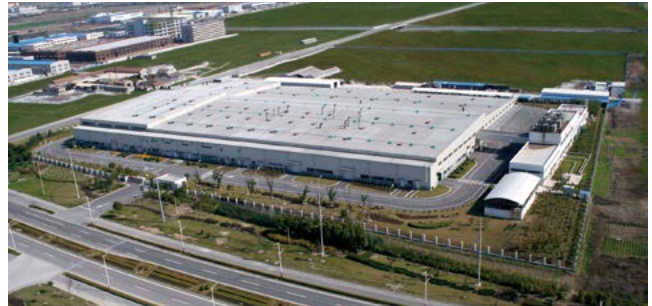
Shanghai Koito Third Plant
