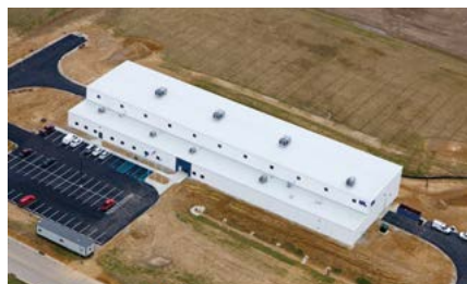
NAL Indiana Tooling Plant
