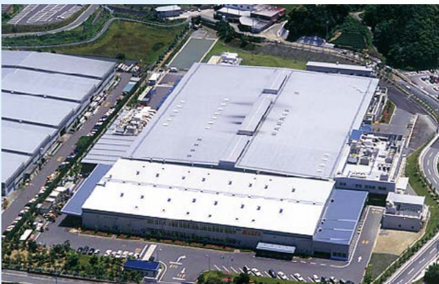
KOITO MANUFACTURING Sagara Plant
