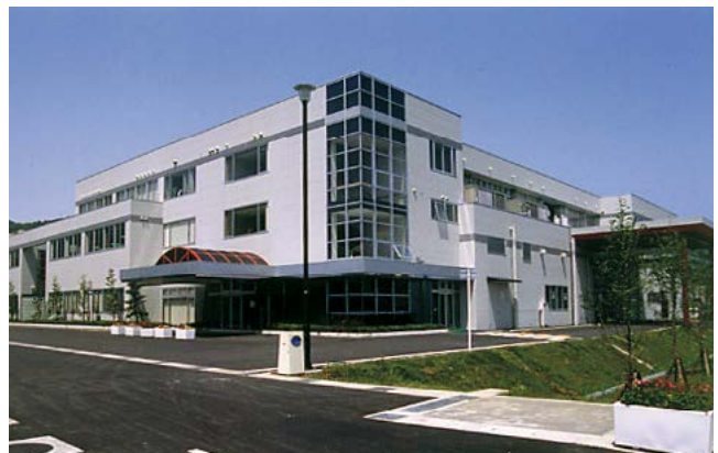
KOITO MANUFACTURING Fujikawa Tooling Plant
