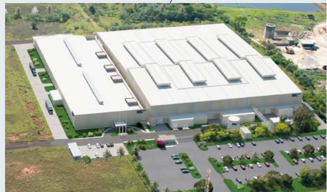
NAL Brasil (under construction)
