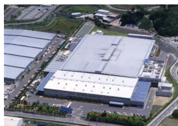
KOITO MANUFACTURING Sagara Plant
