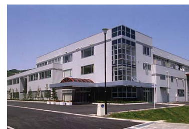
KOITO MANUFACTURING Fujikawa Tooling Plant
