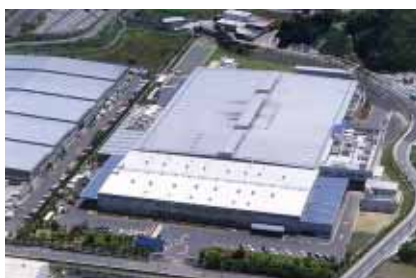
KOITO MANUFACTURING Sagara Plant
