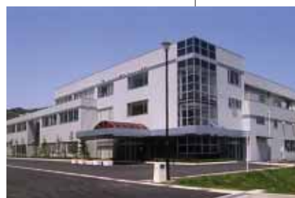
KOITO MANUFACTURING Fujikawa Tooling Plant
