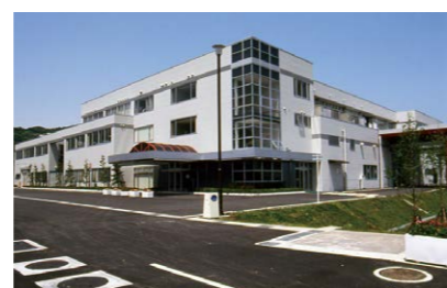
Fujikawa Tooling Plant
