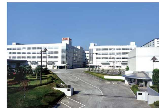
KOITO ELECTRIC INDUSTRIES Head Office and Fuji Nagaizumi Plant
