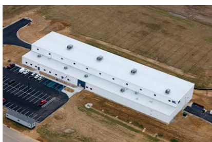
■ NAL Indiana Tooling Plant
