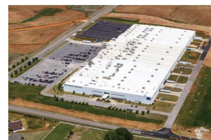
■ NAL Alabama Plant
