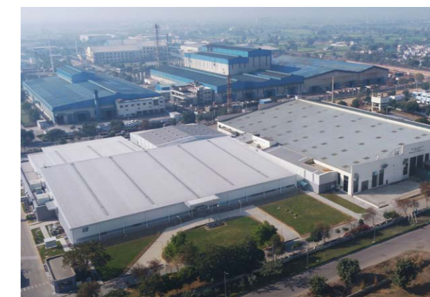
IJL Bawal Plant
