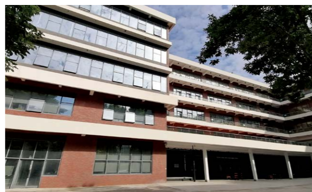
GUANGZHOU KOITO Technical Center (scheduled to commence operations in September 2022)
